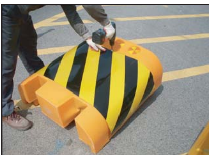
⑩ Attach the reflective on nose plastic tank
