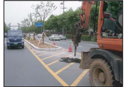
③ Excavation work
