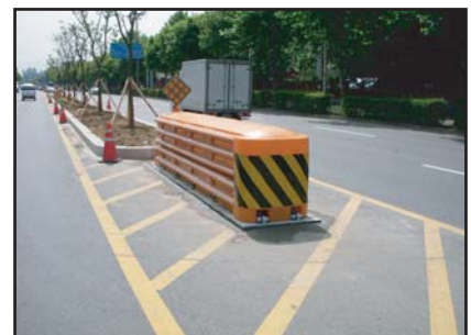
⑫ Complete installation
