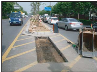
⑤ Complete digging up
