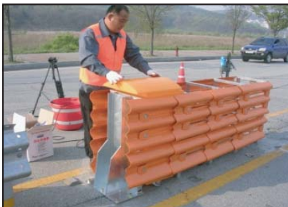
⑦ Put the plastic middle tank
