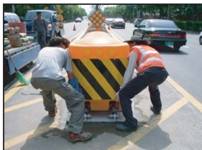
⑪ Assemble nose plastic tank
