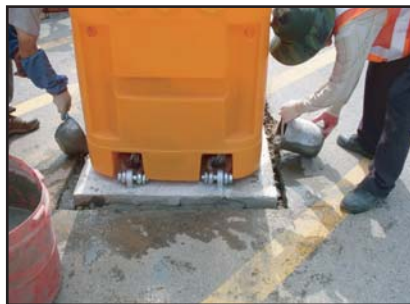
⑧ Fill up the crack by epoxy
