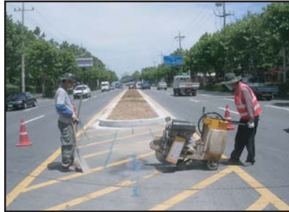
② Mark and cut the road
