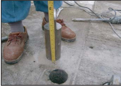
① Boring the concrete for nose holding pin
