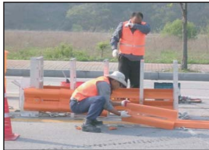
⑤ Assemble the lower part guardrail beam
