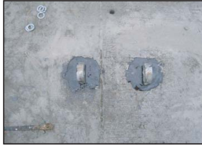
② Fix the holding pin by epoxy
