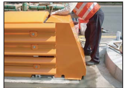
⑨ Assemble the steel back cover
