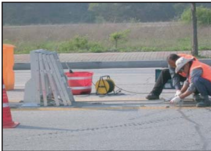
④ Assemble the iron wire and framework
