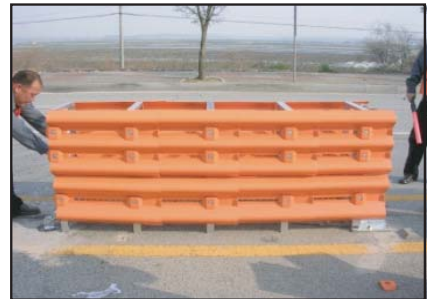
⑥ Assemble the upper part guardrail beam
